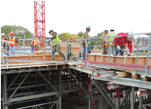
Construction Site and Temporary Office
